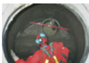
Brønd under renovering.
